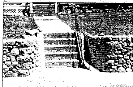
Cobblestone retaining wall
