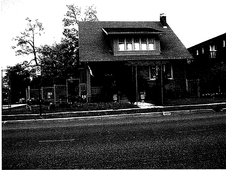
Front of Building on 1100 East
