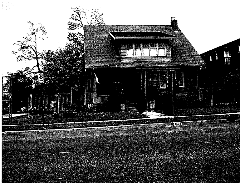
Front of Building on 1100 East
