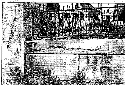
Sandstone retaining wall
