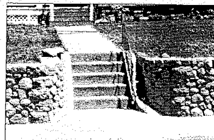
Cobblestone retaining wall
