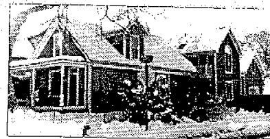
Appropriate: If an addition must be larger, it should be set apart from the historic building, and connected with a smaller linking element, as this one is.
