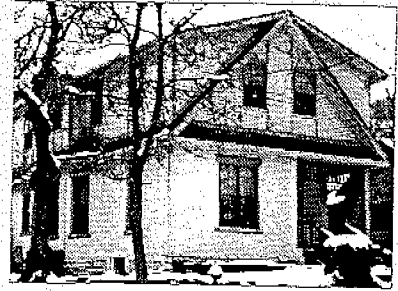
Inappropriate: Keep rooftop additions back from the front of the building or structure.
