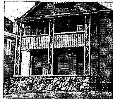
This porch has been altered. As a result, the historic character is compromised.
