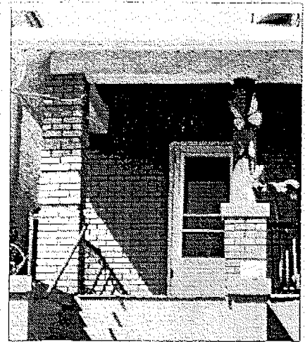
The replacement post on the right is out of character with this house style.
