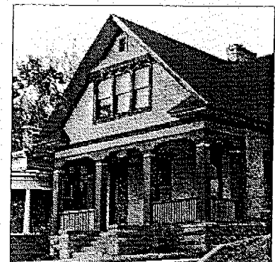
Square posts are distinct features of this inset, full-width porch.
