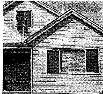
Replacement windows that do not match historic dimensions are inappropriate
