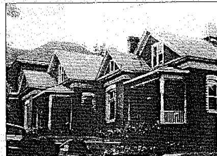
Staggered setbacks in the Marmalade district are due to its diagonal street pattern.
