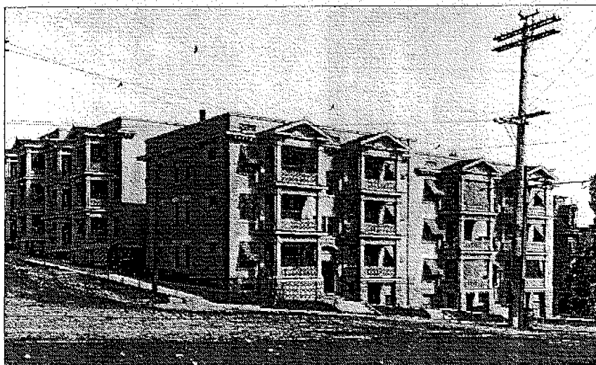
The Kensington Apartments were constructed about 1905, and represent a type of apartment known as a "walk-up."
