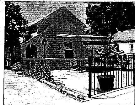
Chain link fences are not allowed when visible from the street.
