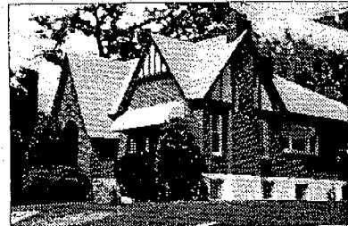
Roof pitches may vary from block to block. The roof on this Tudor Revival house is very steep.
