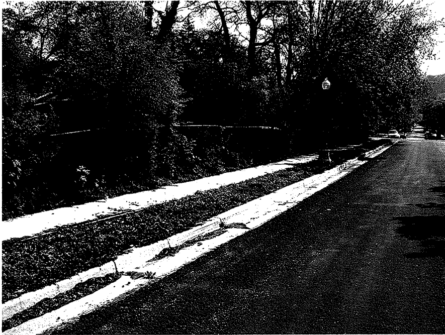
Roosevelt Ave. Looking East Toward 1100 East
