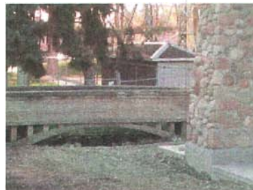
Figure 3: Concrete pedestrian bridge.
