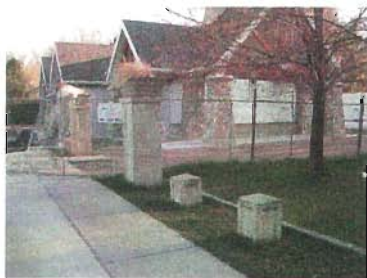
Figure 2: Concrete column planters and bollards. New concessions building behind.
