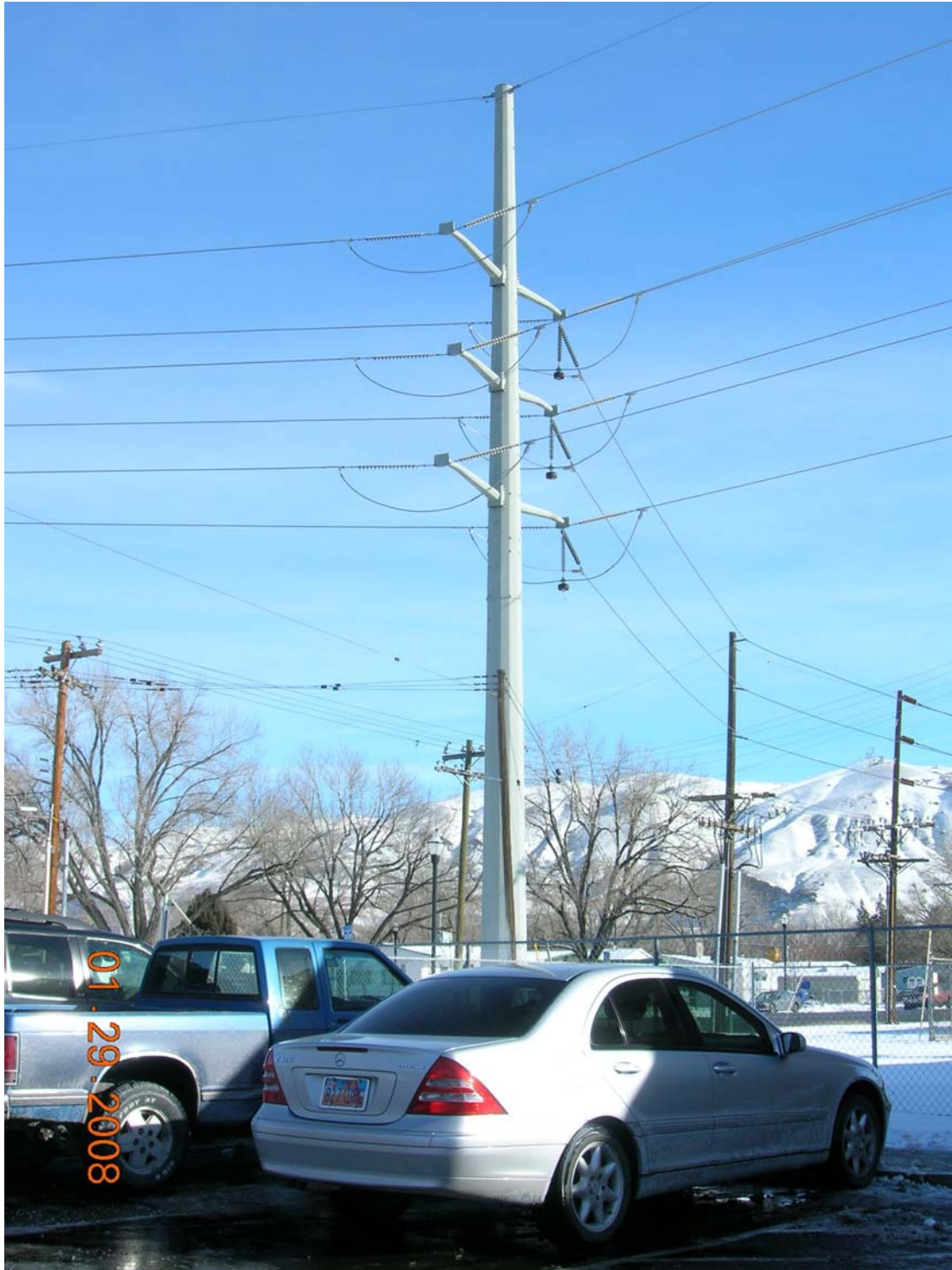
Typical 138 kV double-circuit steel angle structure with line tap.
