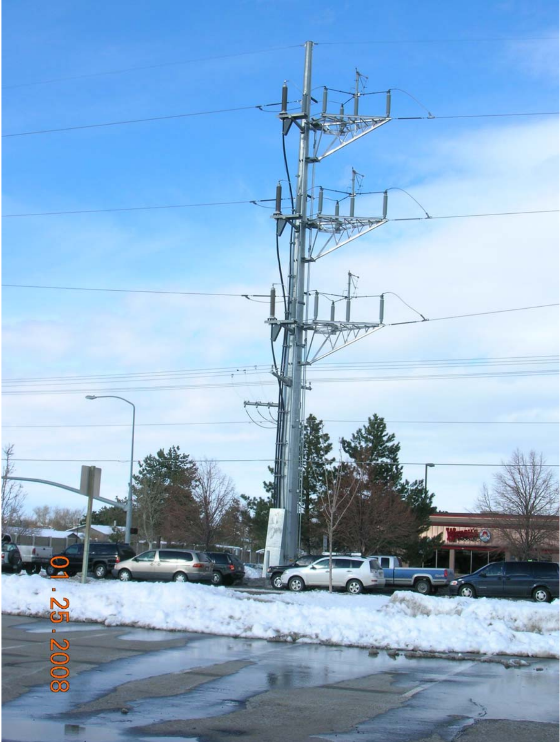
138 kV switch structure with 138 kV underground and overhead lines, 9400 South 2000 East. These structures are typically 80-100 feet tall. This is not a dead-end structure. Two switch structures will be required for McClelland-Emigration: one each at the University and VA taps, 1500 East and 1750 East Sunnyside.
