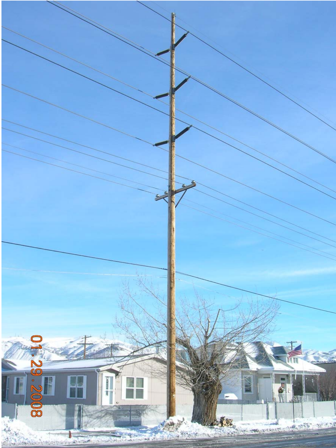
Typical 90 foot wood double-circuit 138 kV tangent structure with distribution.
