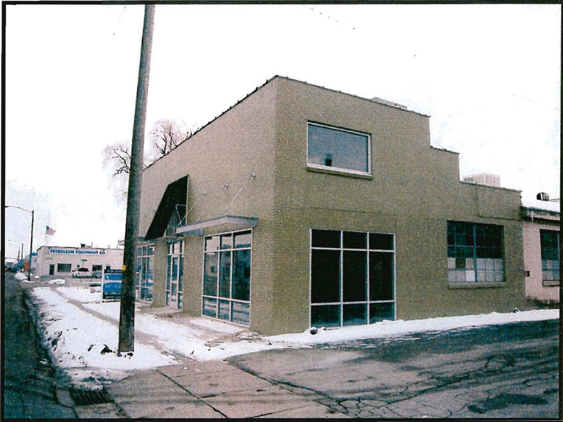
Northeast Corner of Abutting Property – Looking Toward Southwest
