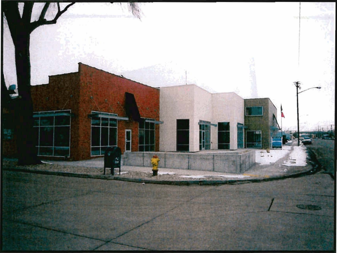
Front Elevation of Abutting Property – Looking Northward
