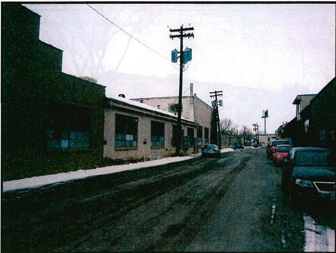
Alley View – Looking Westward
