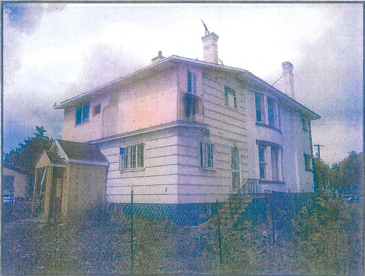
Rear and South Side of Taylor Residence
