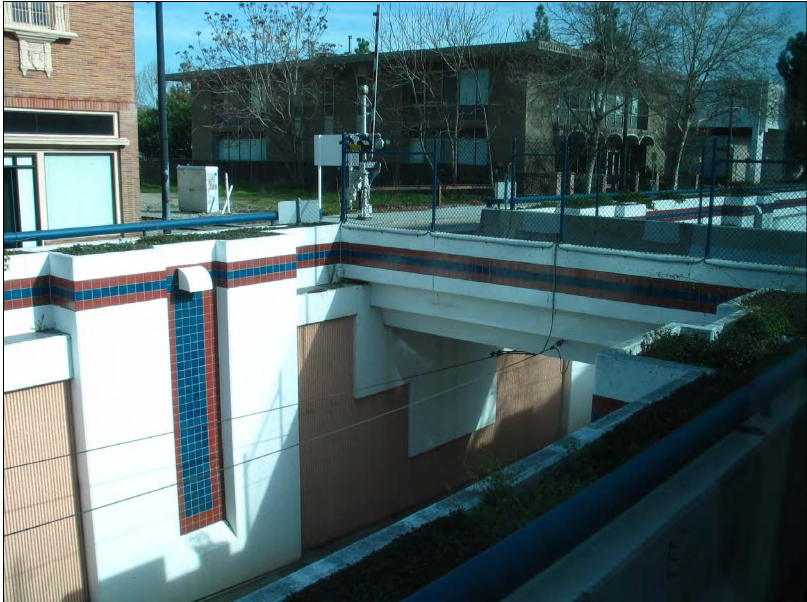
San Jose – Consistent design elements on tunnel under heavy rail line.
