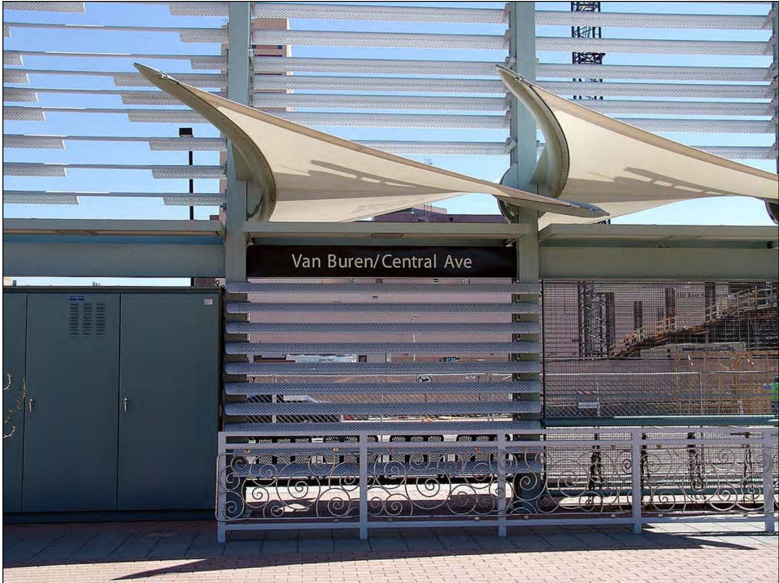
Phoenix – Van Buren/Central station
