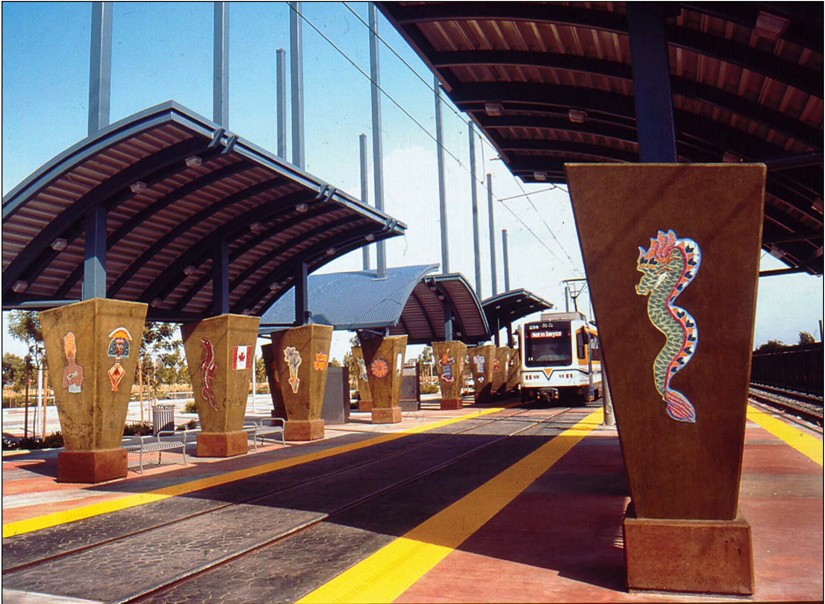
Sacramento – Meadowview station with unique platform supports and paver-embedded track.
