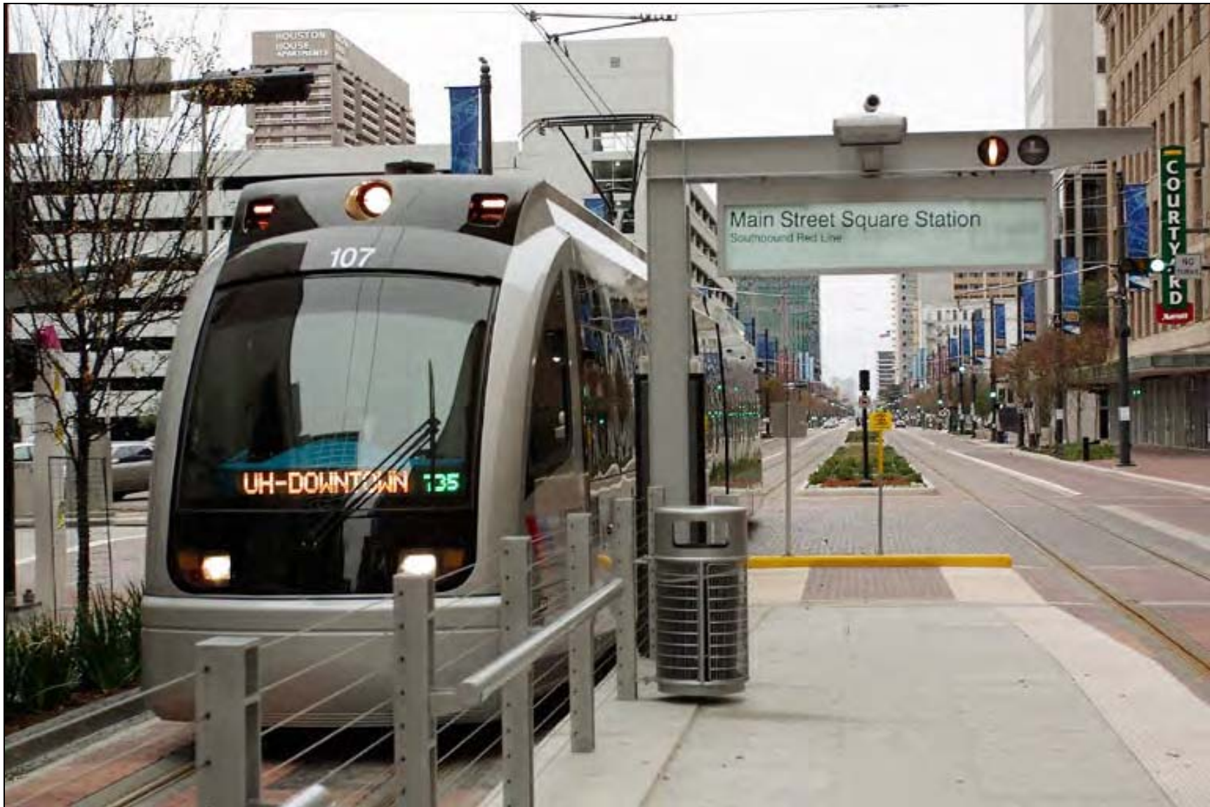
Houston – Main Street Square station with platform elements that reflect train design and establish consistent theme. Brick pavers are used for roadway and track surface.
