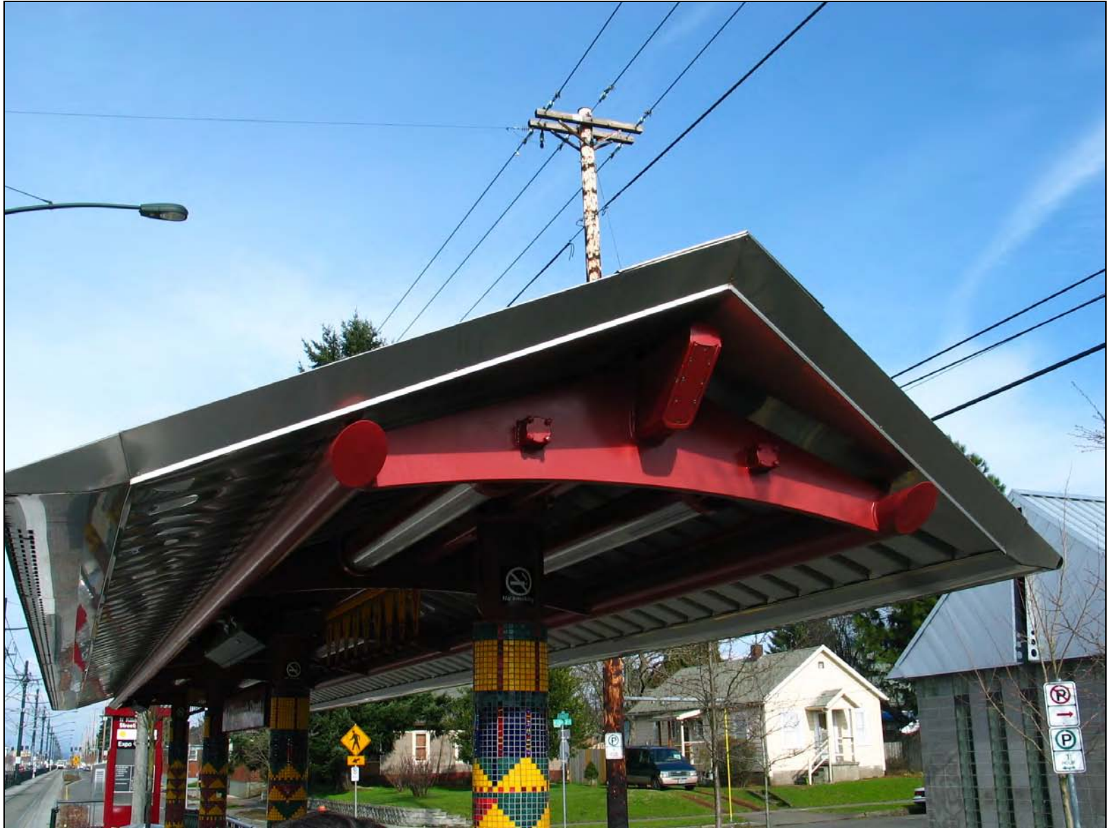
Portland – Killingsworth station with unique canopy and support designs (designed by neighborhood).
