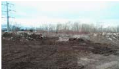
DURING DEBRIS REMOVAL
