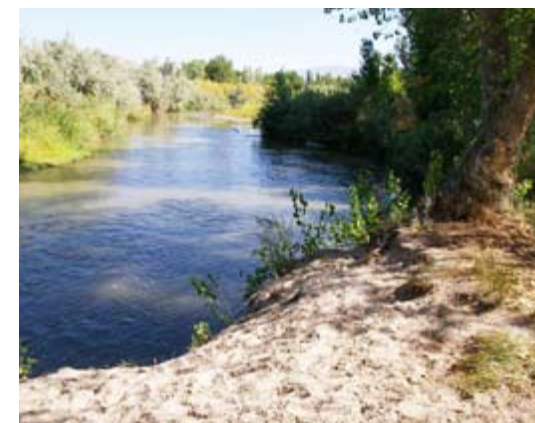
ERODING BANK ALONG THE RIVER
