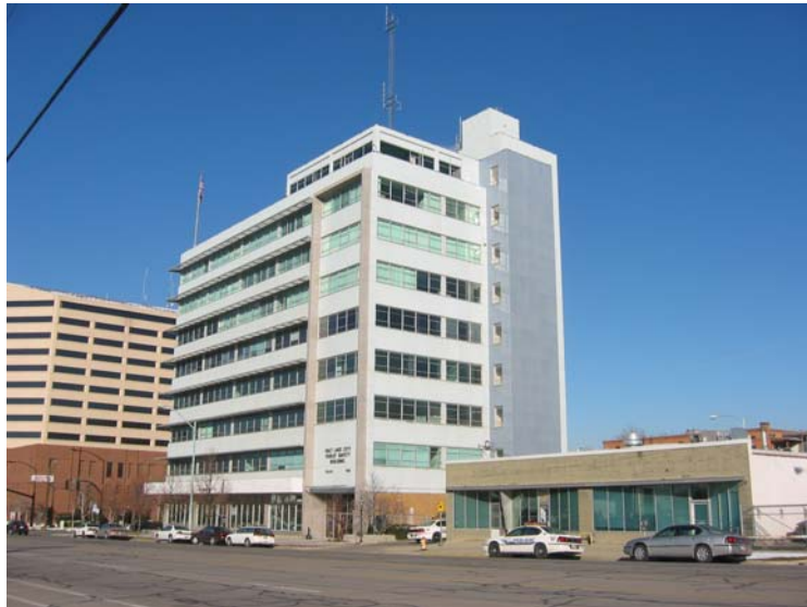
Public Safety Building and Annex Building Street-side
