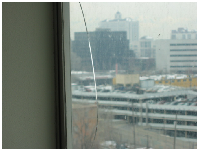
Cracked windows are not regularly replaced
