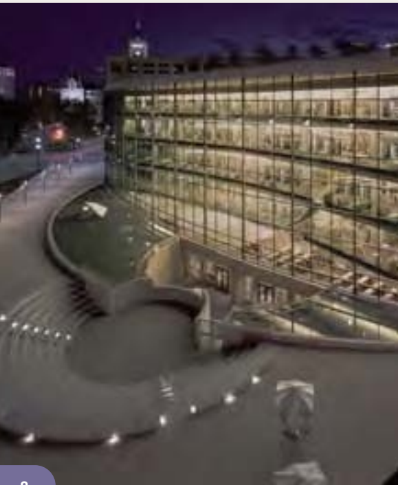
Photo courtesy Big-D Construction
