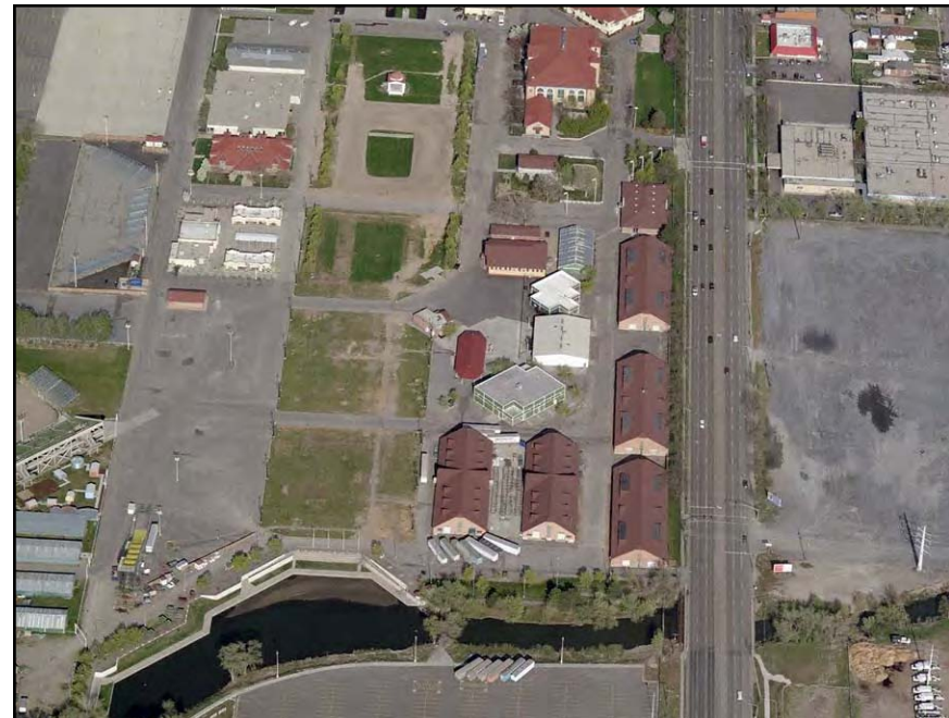
The Utah State Fairpark and the Jordan River looking to the east from the air.
