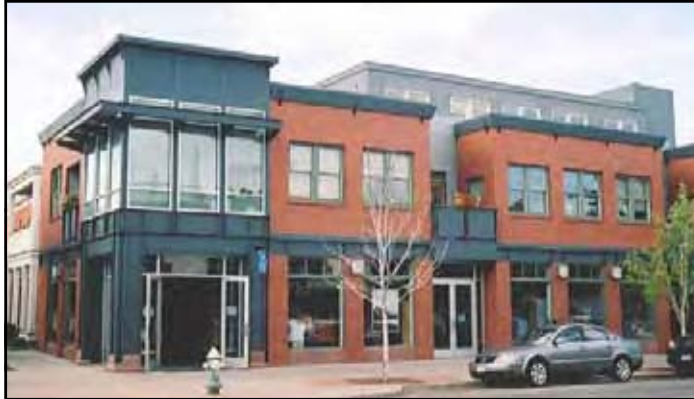
The tallest portion of this building is placed at the corner to make it more prominent.
