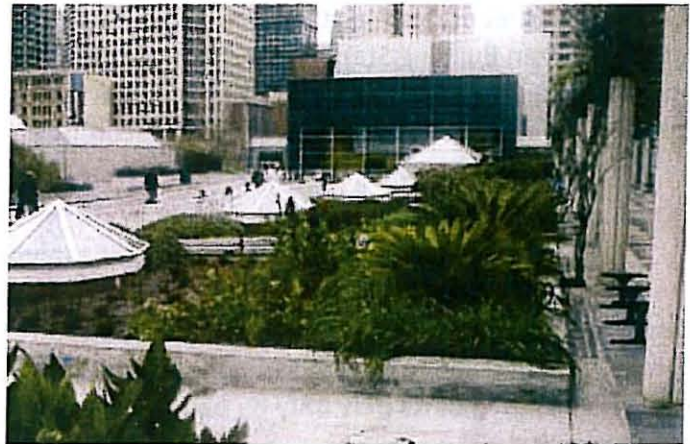
This rooftop garden helps reduce energy costs, reduces storm water runoff and provides places for people to gather.
