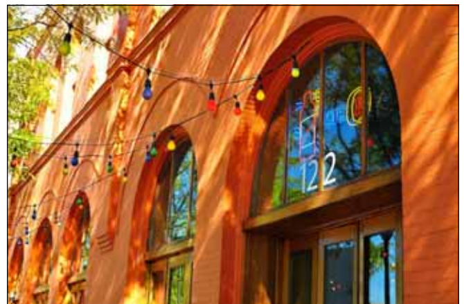
The life of historic buildings can be prolonged by regular maintenance and finding new uses to occupy the space.
