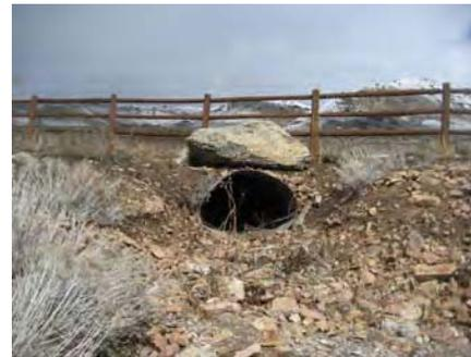
Photo 14: Outlet of third 48" Culvert.
