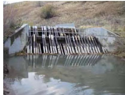
Photo 5: Debris structure at west culvert inlet.
