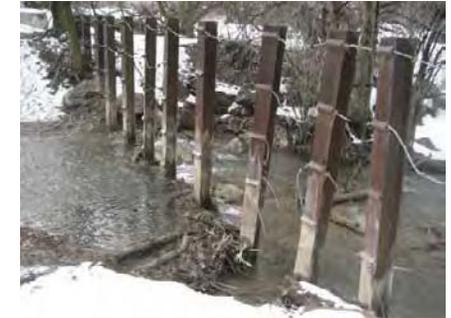
Photo 4: Debris structure west of main bridge.
