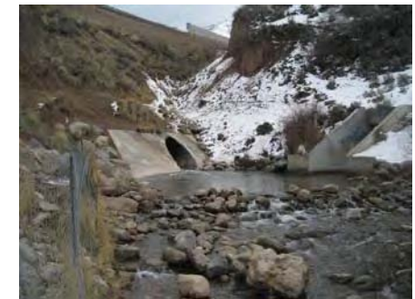
Photo 15: Outlet of Parley's Creek culvert (left side), highway drainage culvert (above it) and outlet of Terminal Reservoir (right side).
