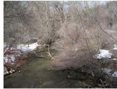
Photo 3: Debris in creek downstream from the bridge.
