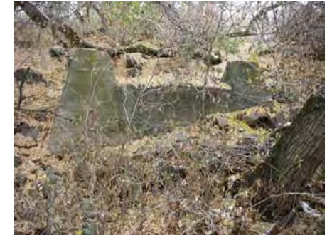
Photo 25: Remnant foundation from gravel and concrete operations.
