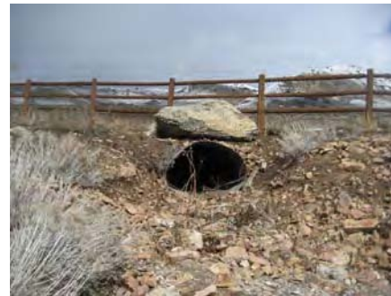
Photo 14: Outlet of third 48" Culvert.
