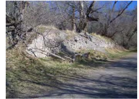
Photo 23: Rock wall lining the historic road.
