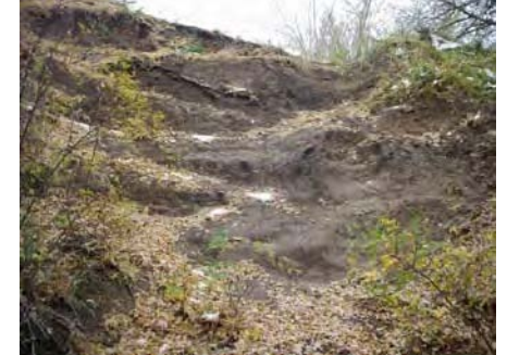
Photo 19: Bank erosion adding sediment to the creek.
