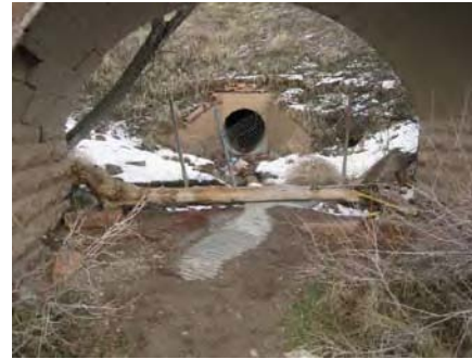
Photo 12: Two culverts for routing off-site runoff through the park. The top of the second, buried corrugated metal pipe is visible inside the archway.
