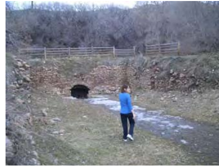
Photo 22: Dudler's Inn cellar and foundation.
