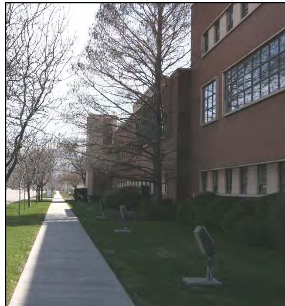
The Rocky Mountain Power office building is typical of an office building found in a Mixed-Use Employment Center station area.
