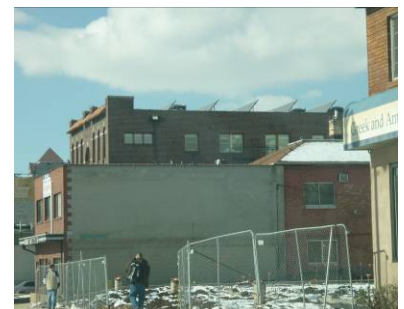
(top) Solar panels in a west side neighborhood. Additional design guidelines could help minimize the profile of such panels in historic districts.
