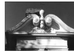
Features such as window hoods, brackets and columns are often associated with particular styles and therefore their preservation is important.
