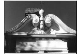
Features such as window hoods, brackets and columns are often associated with particular styles and therefore their preservation is important.
