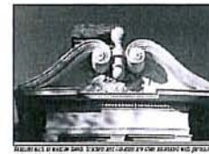
Architectural details help establish a historic building's distinct visual character. Thus, they should be preserved whenever feasible. If architectural details are damaged beyond repair, their replacement, matching the original detailing, is recommended.
