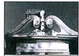
Preserving original architectural details is central to the integrity of the building and its context.
