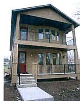
This new house under construction in the Central City historic district is considered a "green build"; however, rehabs can be green, too.
