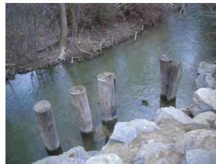
Photo 26: Historic era bridge pylons.
