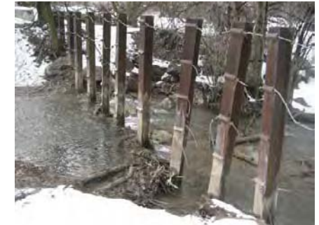
Photo 4: Debris structure west of main bridge.
