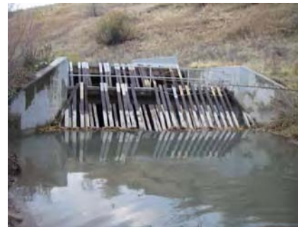
Photo 5: Debris structure at west culvert inlet.
