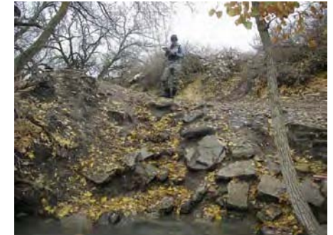
Photo 17: Bank hardening from trail and rip-rap.
