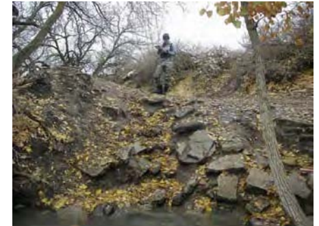
Photo 17: Bank hardening from trail and rip-rap.
