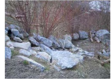
Photo 13: Outlet of Mary's Spring through culvert 2.
