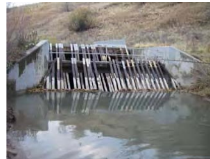
Photo 5: Debris structure at west culvert inlet.
