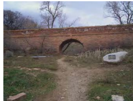
Photo 24: Sandstone aqueduct and foundation.
