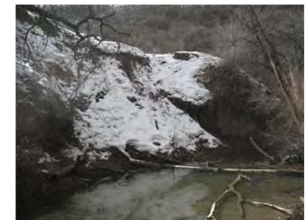
Photo 6: Erosion and debris in channel.
