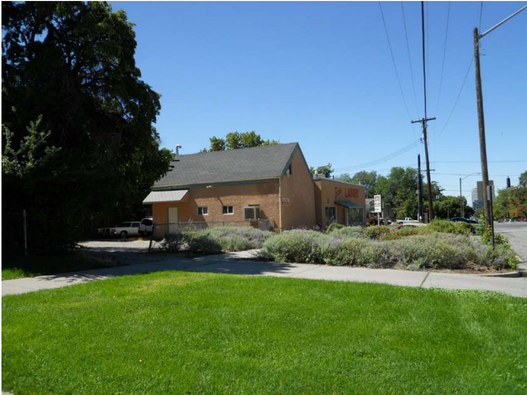
300 South (looking west from driveway)
